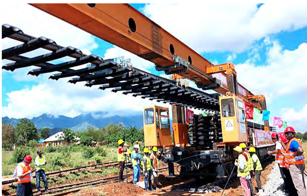
Staff members work at a site of Tanzania's Central Railway Line rehabilitation project undertaken by China Civil Engineering Construction Corporation in Tanzania, April 15, 2019.
