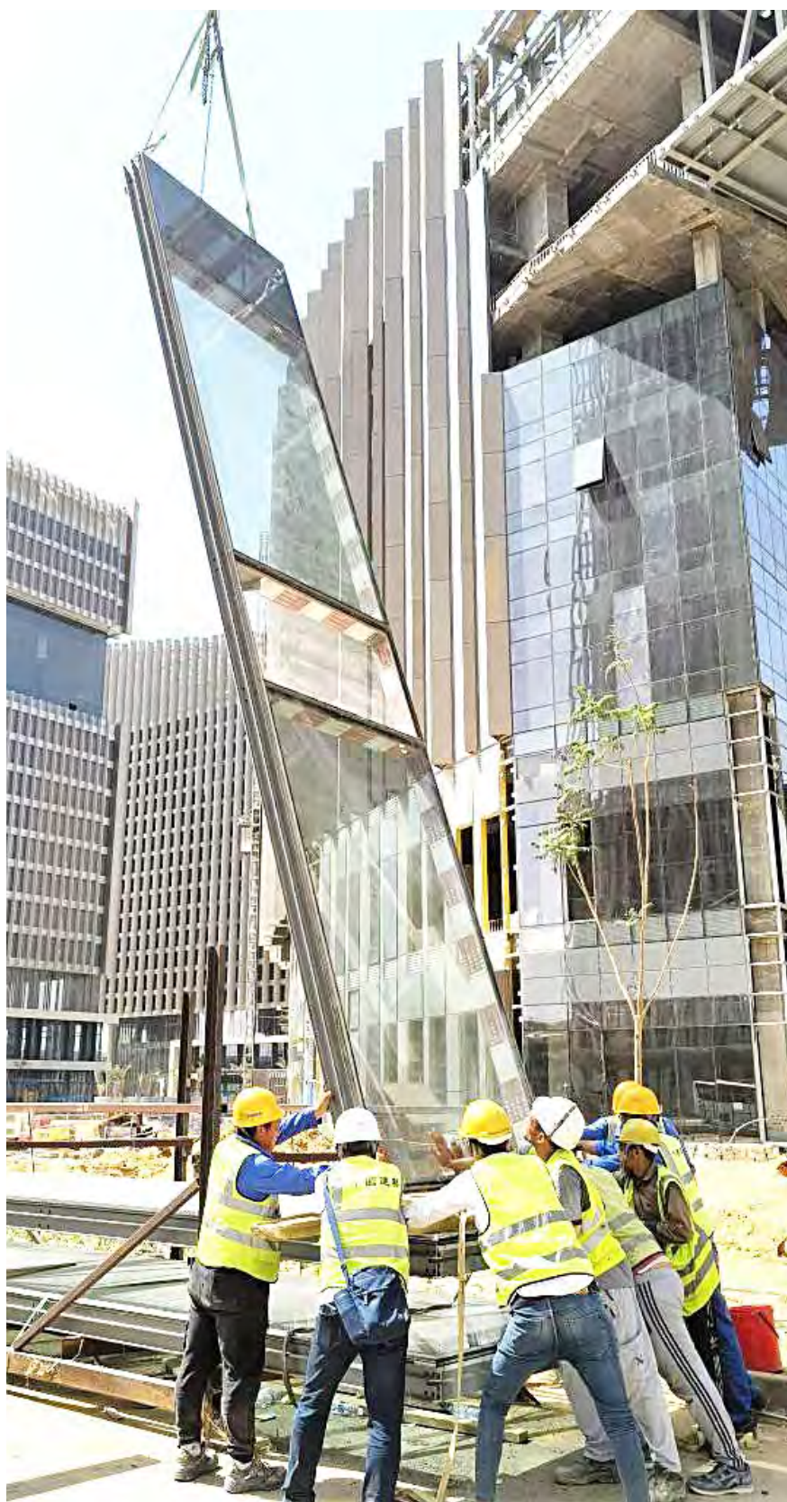
This cellphone photo taken on June 4, 2023 shows workers carrying out hoisting work of the curtain walls at the Central Business District (CBD) of Egypt's new administrative capital, 45 kilometers east of Cairo, Egypt. In the vast and scorching desert in North Africa, Chinese and Egyptian workers are working against the clock to dress up a cluster of newly erected high-rises in glass walls made in China.
